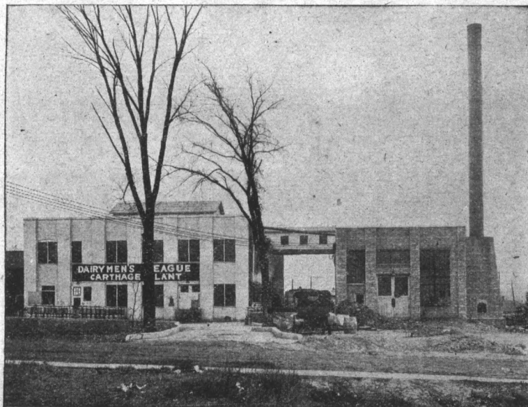
Dairymen's League plant at Carthage, N. Y. This building was formerly used as a factory but was entirely remodeled under the direction of the League's own engineering department. It is one of the best equipped shipping and manufacturing plants which the association owns. During the present season this plant is turning out over 1500 gallons per day of the popular League ice cream.
