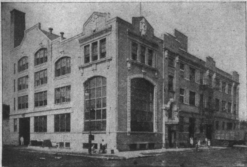
Big distribution plant of the Dairymen's League Cooperative Association at Avenue B and 19th Street, New York City. This modern distribution plant located in the heart of the metropolis was purchased by the League and taken over on September 1, 1922. A large part of the pooled milk of the association goes direct to this plant in New York, from which it is delivered to the wholesale and retail trade. When they are not busy distributing milk the big trucks connected with this plant, are delivering cases of "Dairy-leaf" evaporated milk, which is the brand name recently adopted by the association for this product.
