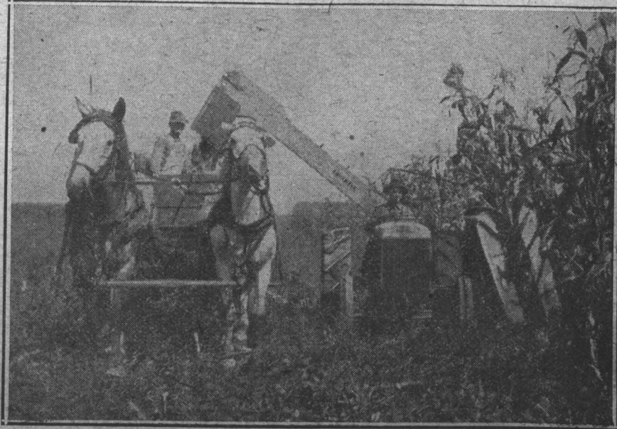
FROM FIELD TO SILO—Ronning ensilage harvester, drawn by a tractor cuts the corn and delivers it as ensilage direct to the wagon hauled alongside. This shows the outfit at work on the Detroit Creamery Company farm in Macomb County, Mich. Mr. Schultz, manager of this farm gives his opinion of its operation on page 19 of this issue.
