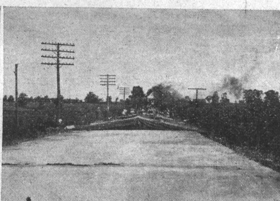
Covering the newly laid concrete with canvas to protect it from the hot sun. The best engineering practices are employed by the state.
