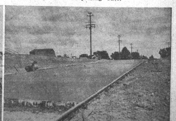
Sketch of partially completed highway at Farmington on the state highway, M-16, showing the detachable steel curbing which is removed.
