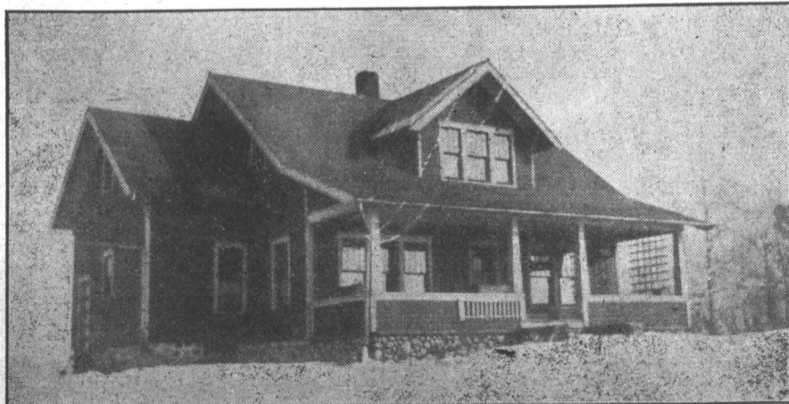
HOME OF MR. AND MRS. EMIL RHODE, MT. PLEASANT, MICHIGAN Mr. and Mrs. Rhode write that their home is a modern eight room bungalow, 26 feet by 32 feet, with an addition, nine feet by eighteen feet, on the west end. The porch is eight feet deep and runs across the entire front of the house. They have furnace, bath, hot and cold running water, and gasoline lights. Woodwork is of hemlock and doors are fir with floors of oak and pine. There is a basement under the entire house, eight and one half feet deep.
