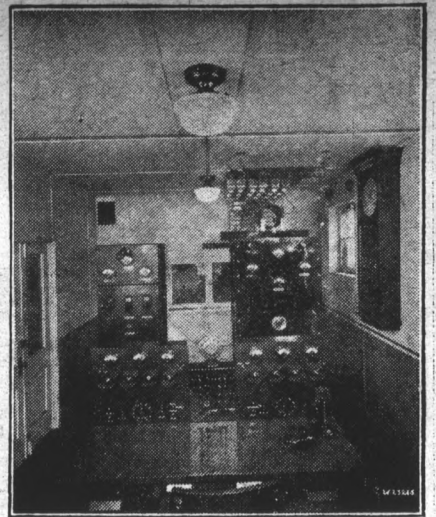
An excellent view of the operating room of radio station WGHP of Detroit.
