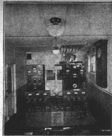
An excellent view of the operating room of radio station WGHP, of Detroit.
