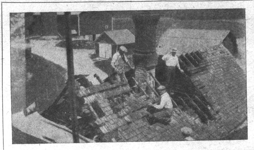
If it had not been for the fact that this roof fire was discovered shortly after it started and a dry powder extinguisher was handy the damage to this home would have been much greater than shown here. Had the roof been fire proof this would never have happened.
