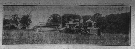
A closeup showing how Mr. Shear mounted his Fordson tractor motor on his combine as a power plant.
