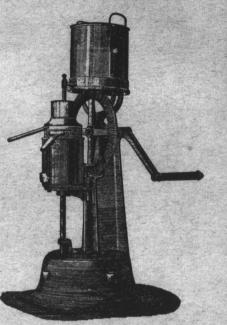
AN EARLY MODEL This cream separator, a De Laval, is an early model, built for hand operation and known as the bevel gear type. Many of our readers will probably recall hav-ing seen or owned one. Some difference between this and the present day type, isn't there?
