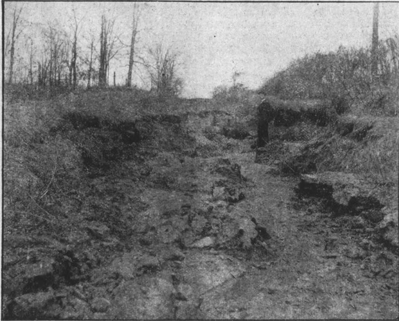
The Ditches by the Side of the Road on this Hill were Allowed to Fill, Causing the Roadway to be Destroyed by Erosion.
