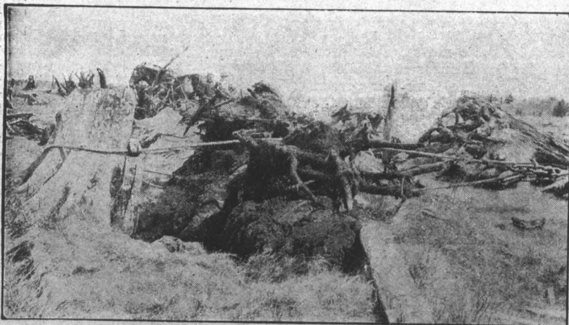
Big Pine Stump Split with Dynamite, One-half of which has been Pulled.
