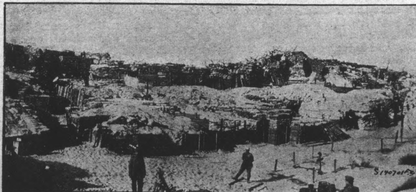
German Trenches on the Seacoast of Flanders Connected with Bomb-proof Shelters Made of Timber and Bags of Sand.
