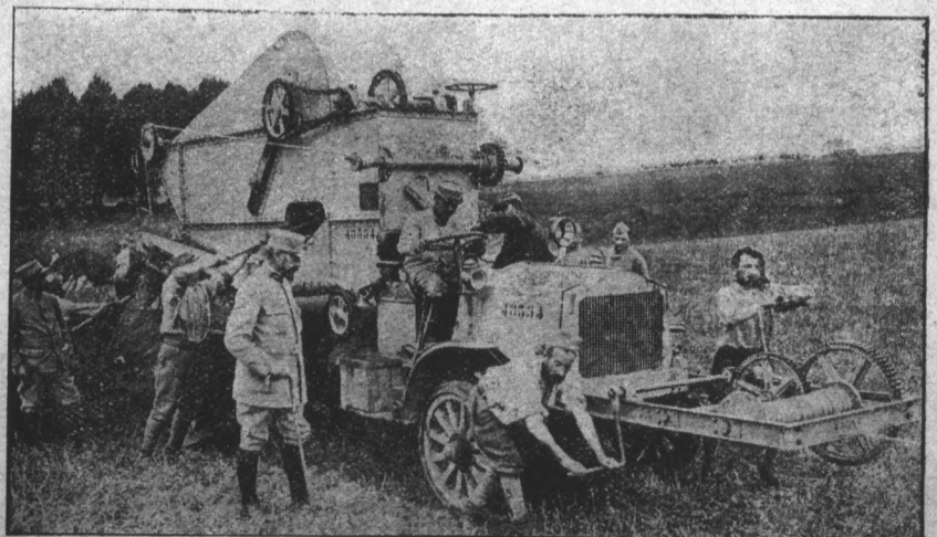
French Tractor Digs Trenches and Constructs Breastworks as it Travels.
