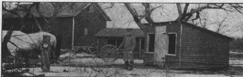
Moving a Colony House on Planks or Skids.
