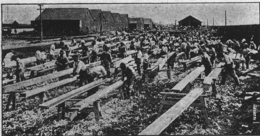
Carpenters at Work on New Hangars at One of American Aviation Schools.
