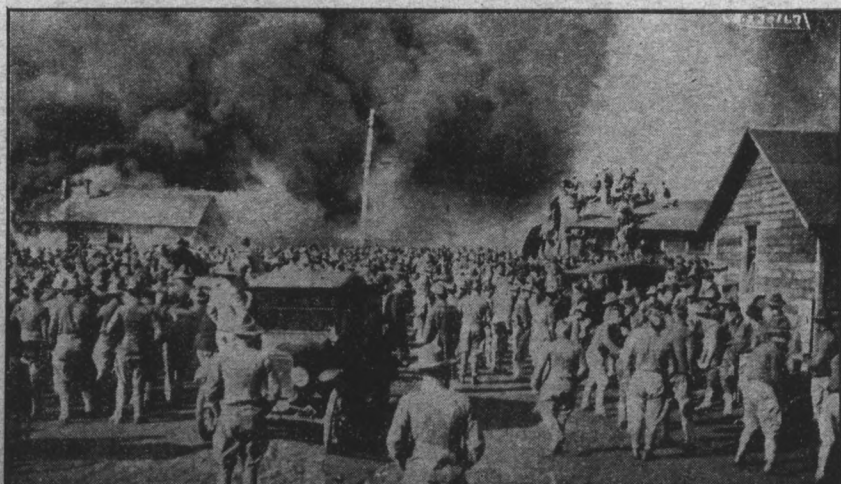
Fire Destroys Soldiers' Quarters and Store Houses at American Army Post.
