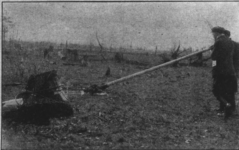
One-man Stump Puller, One of Three Types Used at the Demonstration.
