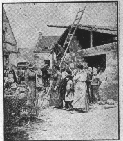
Rebuilding Homes in Reconquered Portions of France.
