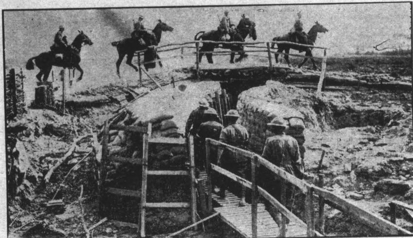
Where Communication Trench Lines Cross Roads, Subways Are Constructed to Prevent Possible Congestion of Troops or Supplies.
