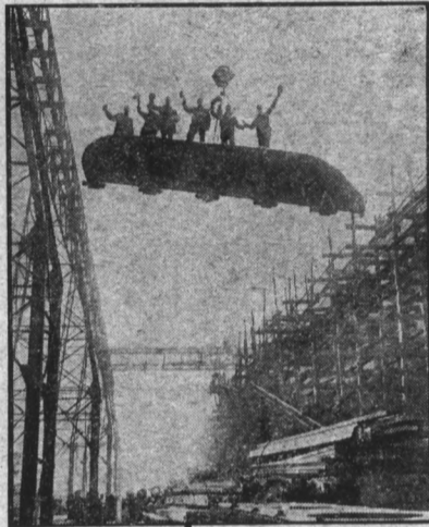
Placing the Mammoth Rudder in One of the "Victory" Ships that America is Now Building.
