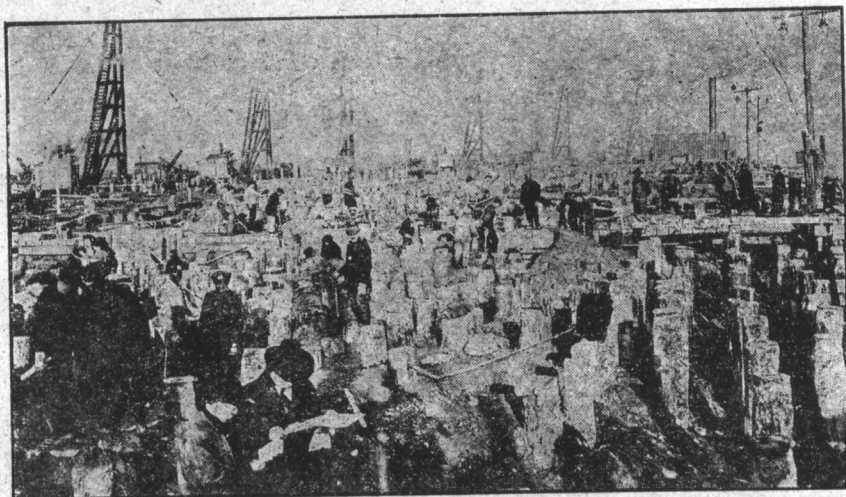
Pile Driving at Extensive Shipyards at Hog Island where Work of Building Ships will be Pushed Rapidly.
