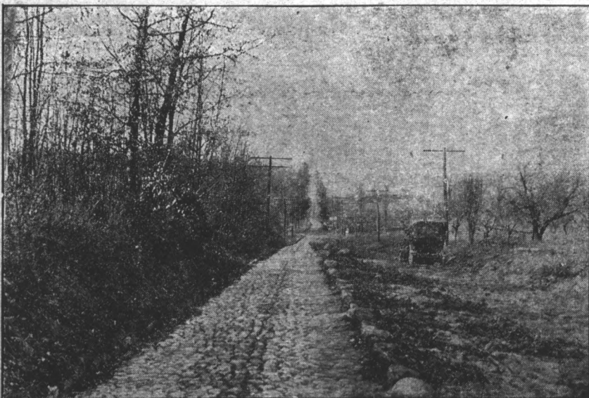
A Long, Steep Sand Hill Paved with Stone Over Thirty-five Years Ago. Not a Stone Ever Became Loose. (See Story on Page 517).
