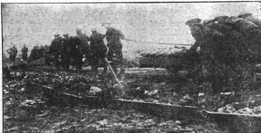
This is how the Tommies get ammunition to their guns at the front, over a line of temporary railroad. The shells on this hand car are for one of the eight-inch howitzers which are doing such effective work.
