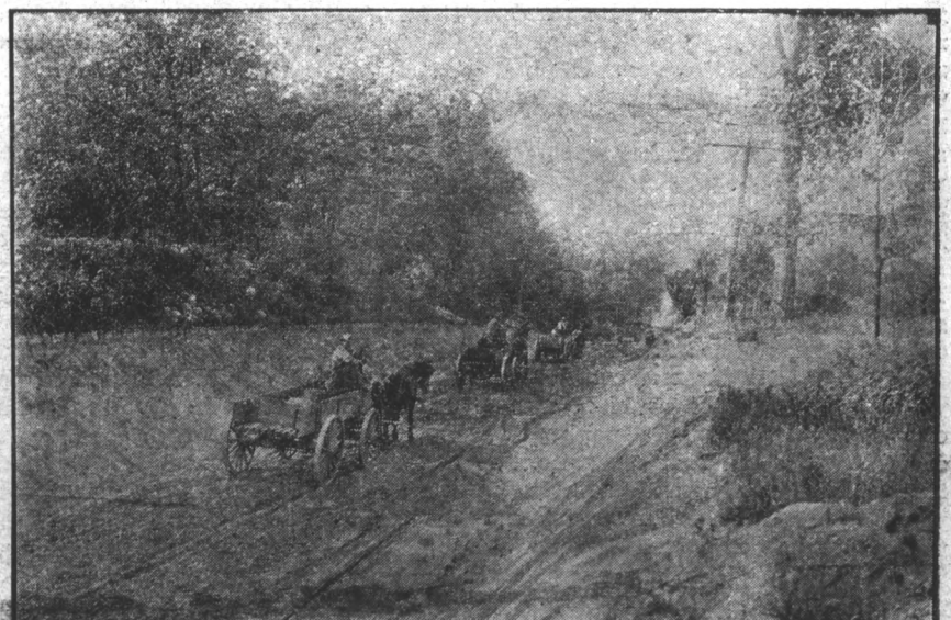
Farmers and Townsmen Removed Paving, Cut to Six Per Cent Grade and Surfaced with Gravel to the Benefit and Delight of both Country and City.
