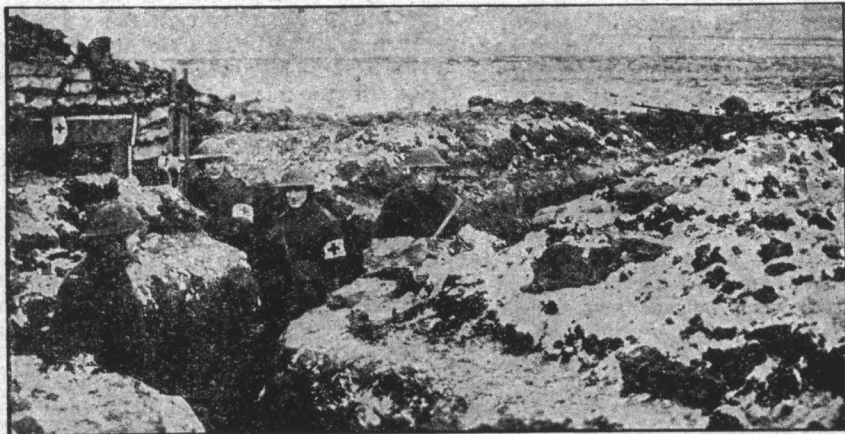
Dugout in a trench held by the American forces, used as a dressing station. These men of one of the medical squads have a stretcher in readiness, while at the right is a trooper keeping guard with a machine gun.
