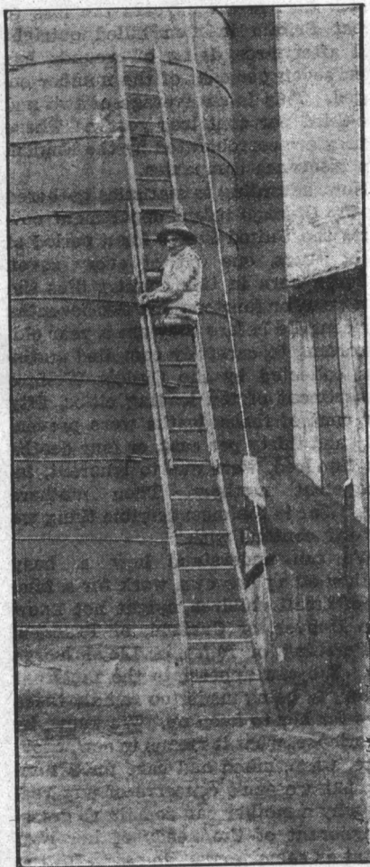
Tightening the hoops on the silo is a task none too difficult for this plucky man.
