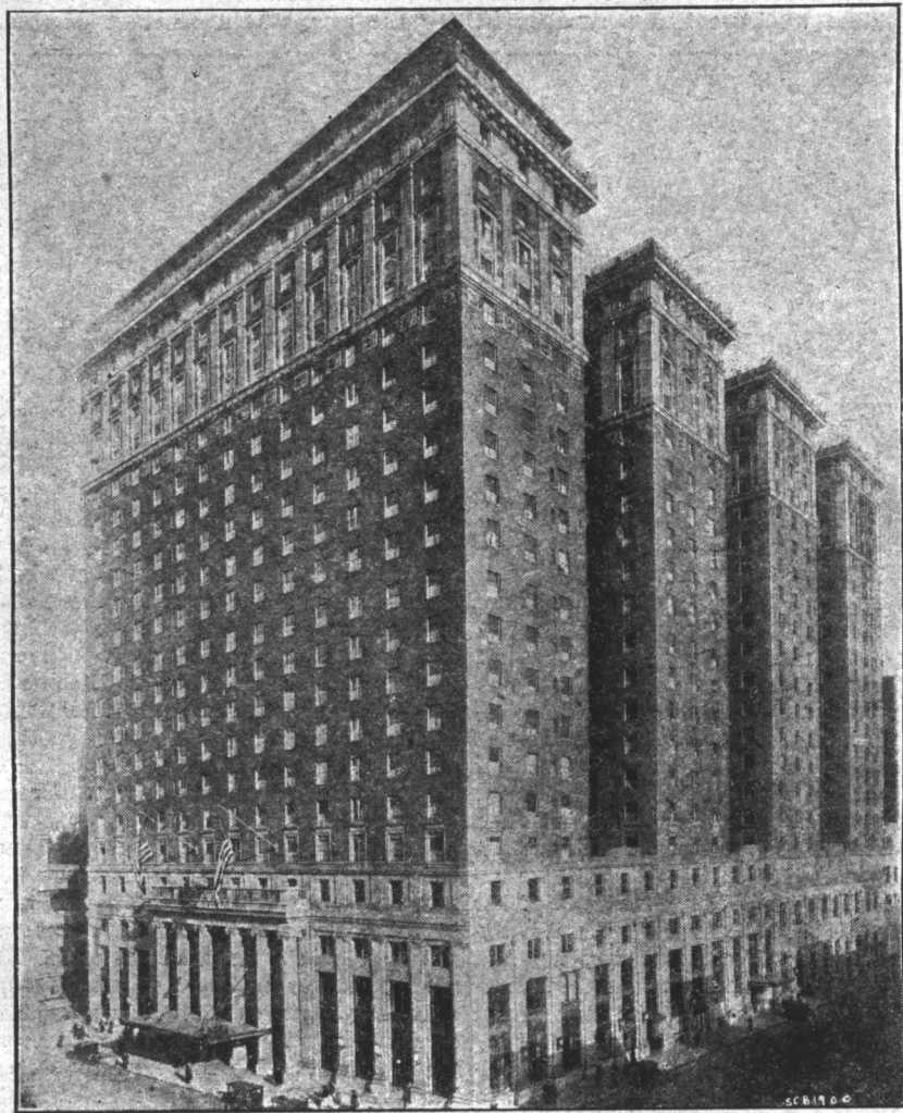
The Recently Opened Pennsylvania Hotel, New York City, is the Largest Hostelry in the World, having a Capacity of 2,200 Guest Rooms. Special Elevators Convey the Guests to the Ball-rooms, or Social Parlors, while Another Operates to the Roof, where one may Dine in an Elegantly Appointed Restaurant, which Affords, from its Elevation, a View of the Entire City.
