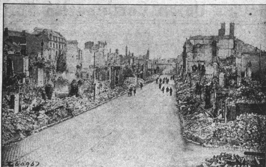
Rheims, France, Destroyed, yet Immaculate. This picture of the Rue Chanzy, Rheims, illustrates the remarkable ability of the French in Renovating Ruined Cities.
