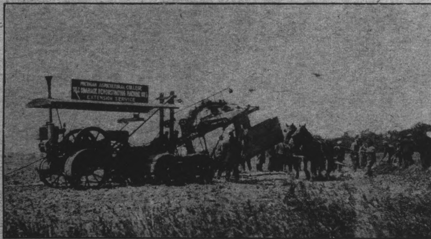
Using Team and Board Scraper in Covering the Tile.
