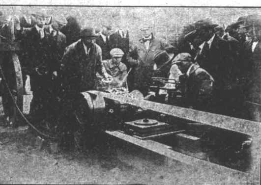
Testing the Belt Power of Gas Tractors.
