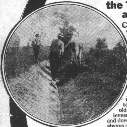
The Martin cuts a "V" shaped ditch down to four feet deep
