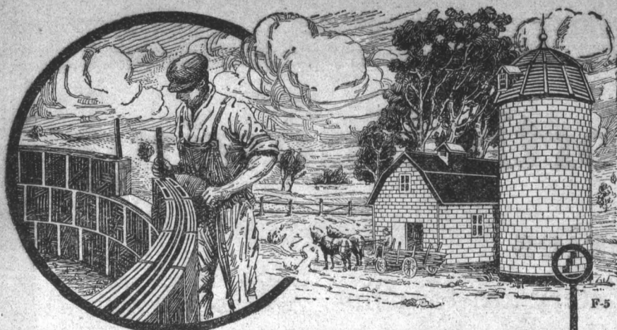
Placing the reinforcing steel of the door opening.
