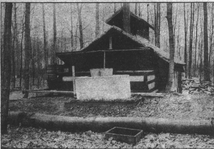
This looks like an up-to-date outfit. Notice the gathering tank with cover and screen cover. The covered storage tank on the north side of the sugar house is another good idea for sap will keep cooler in the shade. One more thing that works well is the keeping of ice in this tank.
