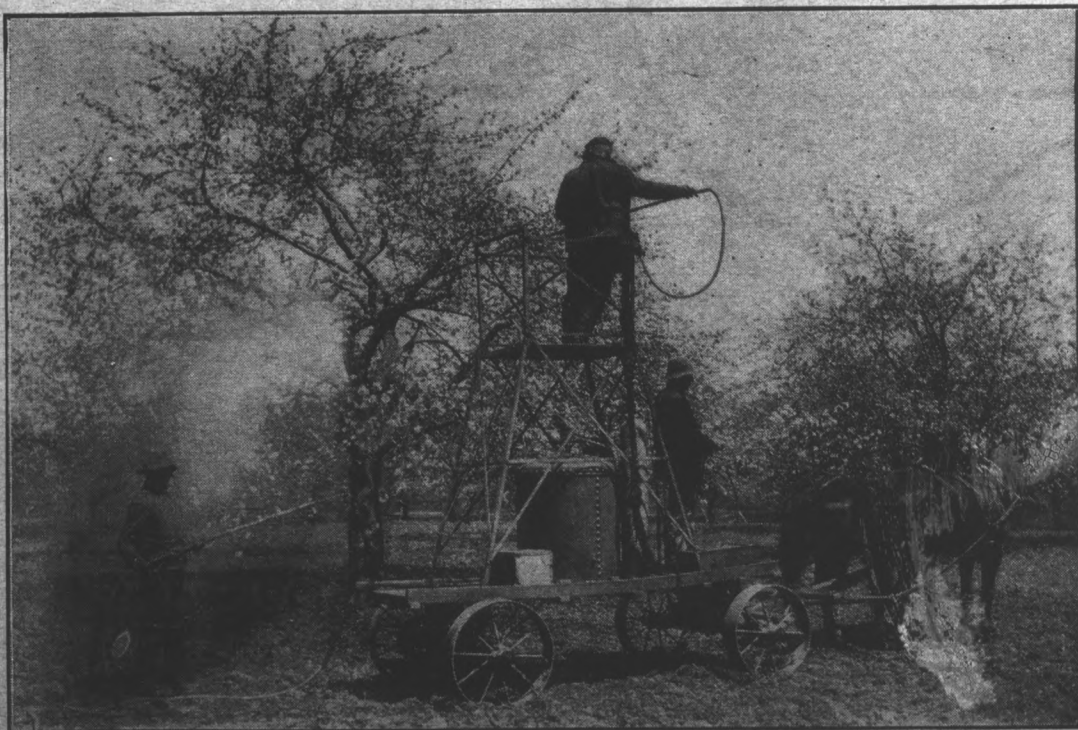
Having a Supply of Water that is Quickly Accessible, Such Jobs as Spraying Are Done in the Minimum of Time.
