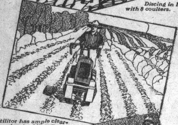
Utilitor has ample clearance for straddle row cultivation.
