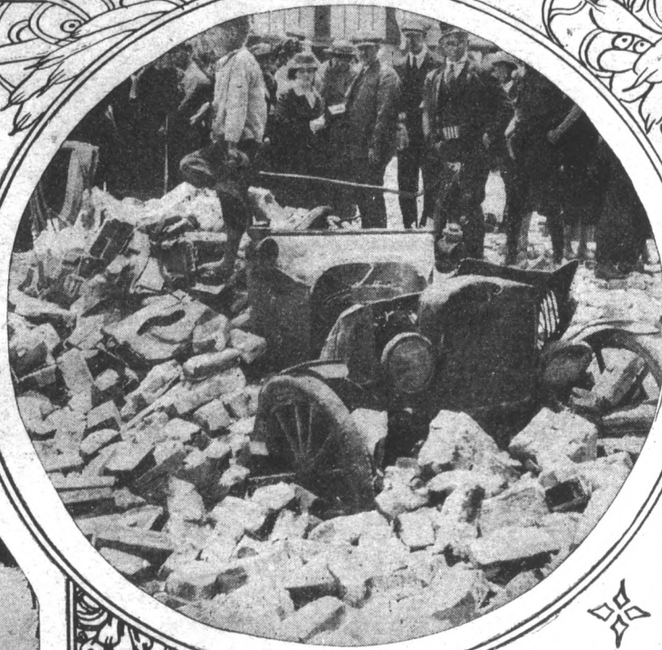
Earthquake shocks at Los Angeles tumbled a brick wall on this automobile, completely wrecking it.
