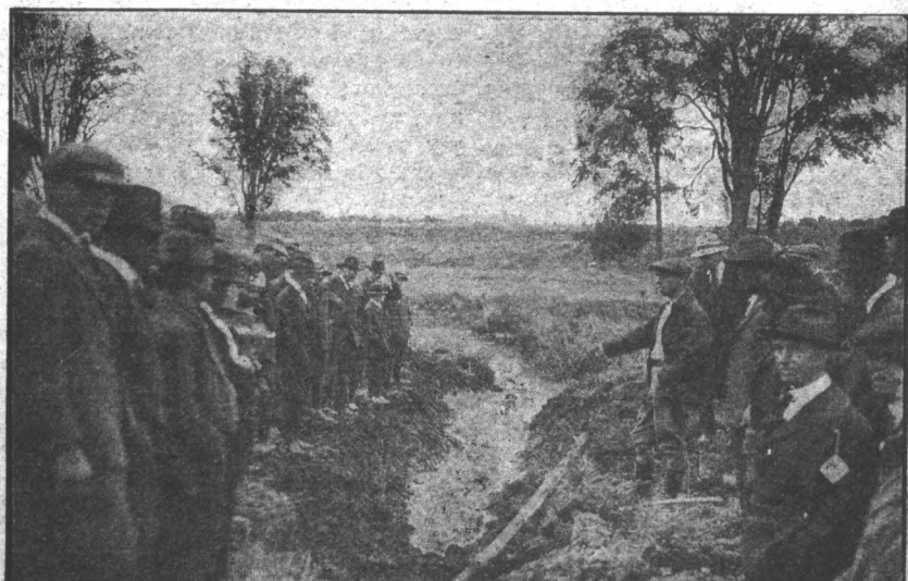
Building Drains with Dynamite Proved a Big Attraction.
