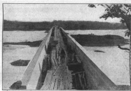
The Shell Above the Arches which was Filled with Gravel and Earth.
