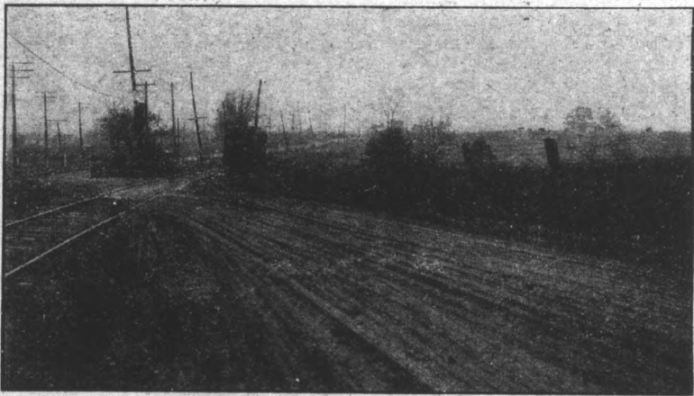
This Dangerous Crossing Near Marshall will Soon be Obliterated by New Right of Way.
