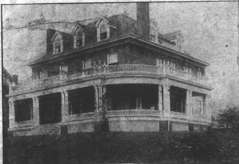
Shrubby and Flowers would Add Greatly to the Appearance of this House, Relieve the Straight Lines, and Make it More Home-like.
