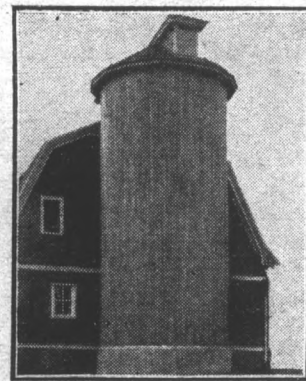
Double wall "home-made" silo. Any species of sound knotted lumber can be used.
