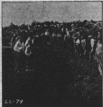
Ditching by the Use of Explosives.
