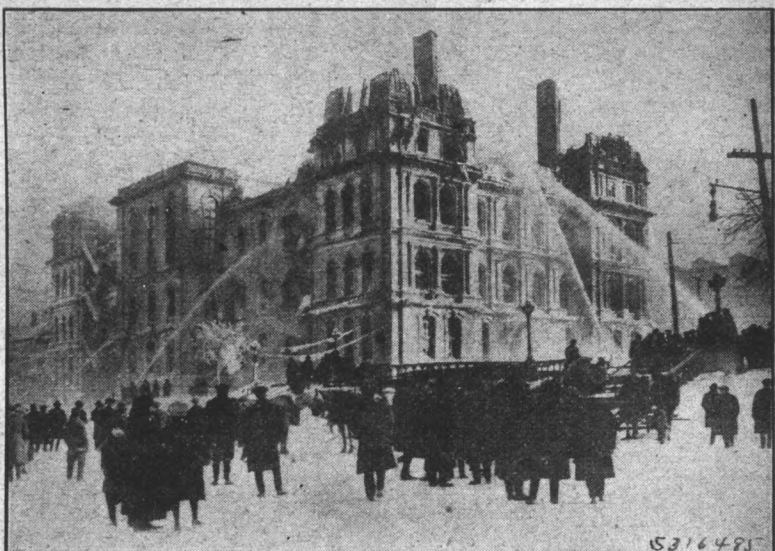
The firemen had to fight cold as well as fire in the ten million dollar blaze in Montreal in which the city hall and valuable documents were destroyed.
