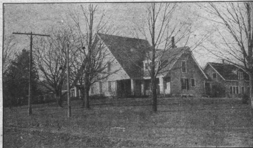
The Homestead Built by Governor Crapo a Half Century Ago still Stands as Convincing Evidence that the Governor Built Well.
