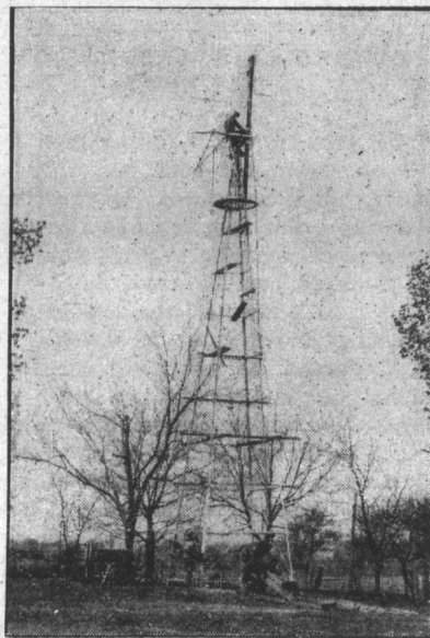
Erecting Wind-propelled Electric Plant on Farm of William Simcoe.
