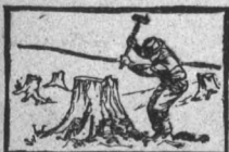
1 Driving the hole
