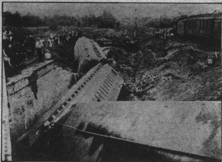
A view of the express train wrecked between Camden and Atlantic City. Twenty were killed and about seventy-five injured when the train plunged down a forty-foot embankment.
