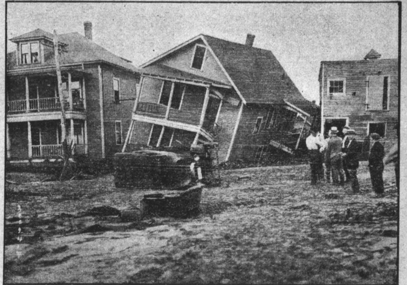
A property loss of $500,000 resulted when the high concrete and earthen dam in Willimansett, Massachusetts, gave way, releasing millions of gallons of water.
