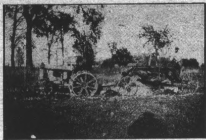
Using the Tractor to Fill Trenches.
