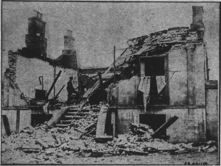
All that was left of the home of M. A. Corrigan, Free State official, at Rathmines, Ireland, after the explosion which had been ordered by the Republicans.
