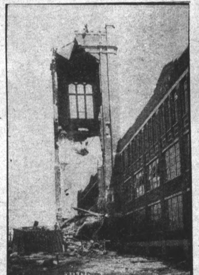
Five men were killed and several injured when this tower collapsed in Hartford, Conn.
