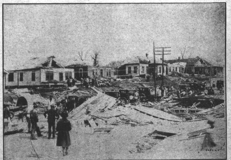
One of the freak characteristics of a tornado which swirled over Alexandria, Louisiana, completely wrecked one building to matchwood, while across the street two small houses were unharmed.
