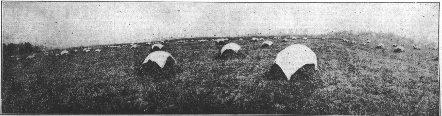
Alfalfa Curing Under Hay Caps on Roycroft Farm, in Houghton Co.—An Example of Success with This Forage Crop in the Upper Peninsula.
