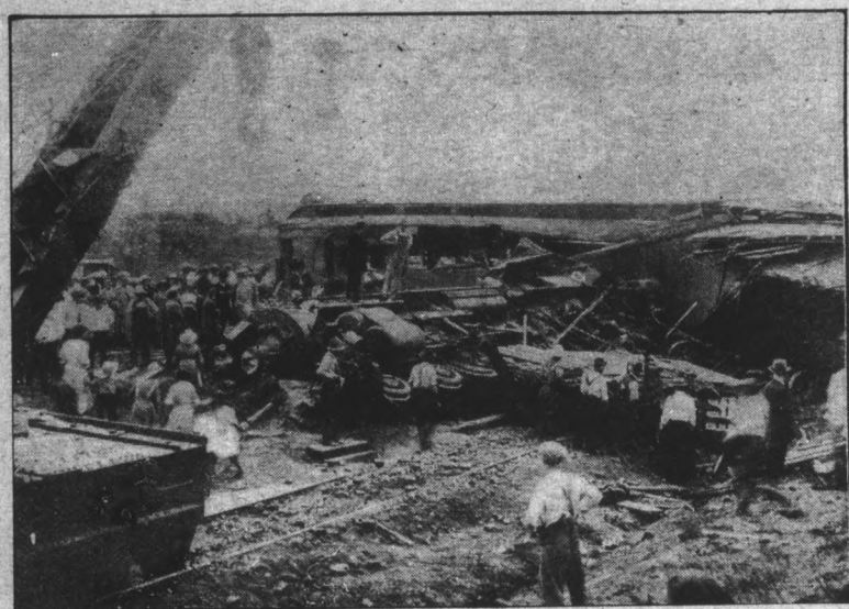
A defective rail is believed to have caused the wreck of the Knight Templars' train at Durand, Michigan, in which five persons were killed and twenty-five injured.
