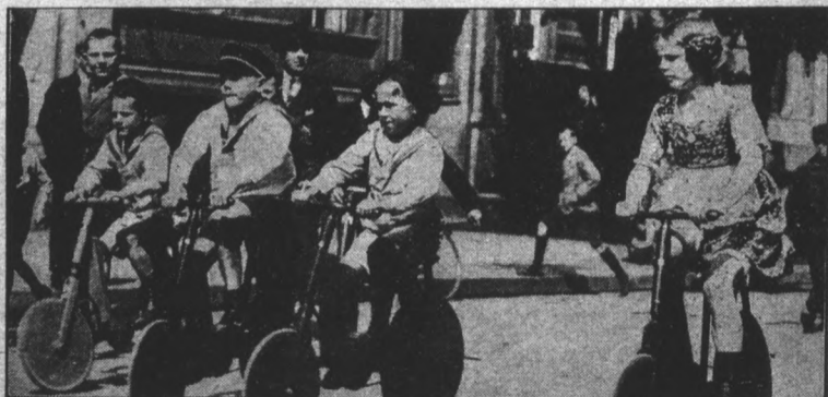
Because steel is too dear, these Berlin kiddies ride wooden bikes constructed mainly of wood, with hard rubber tires on the disc wheels, and a leather belt for the usual chain.
