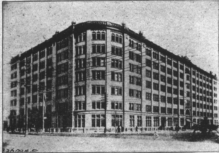
This steel-framed sky-scraper, in Tokio, Japan, built by an American building company, was only one of the many modern buildings which tumbled in Japan's recent quake.
