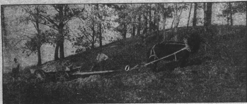
At the Stop Pile Where the Marl will be Left Until Spring.
