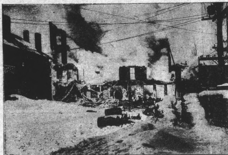
In the heart of Montpelier, Vermont, this fire caused the death of eleven people, with nine injured, and a property damage of $300,000. The flames dangerously threatened the city hall.
