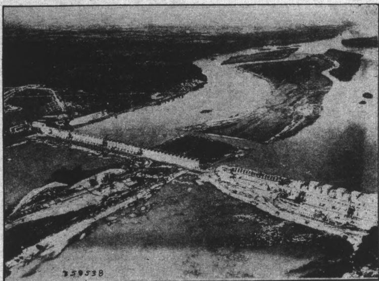
Jackson Island, shown in the center of the river, will be submerged when the Wilson dam is completed in October. It will form a lake 18 miles long and a mile wide.
